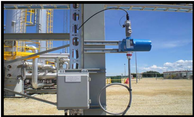
**FIGURE 8: NEMA4X Enclosure and Heater Power Supply**
